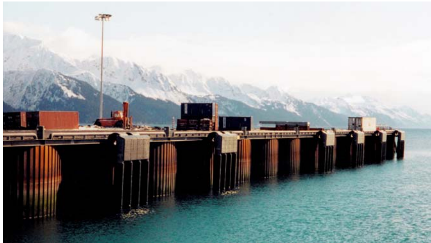
Figure 10. Open Cell Bulkhead Dock with Fenders
