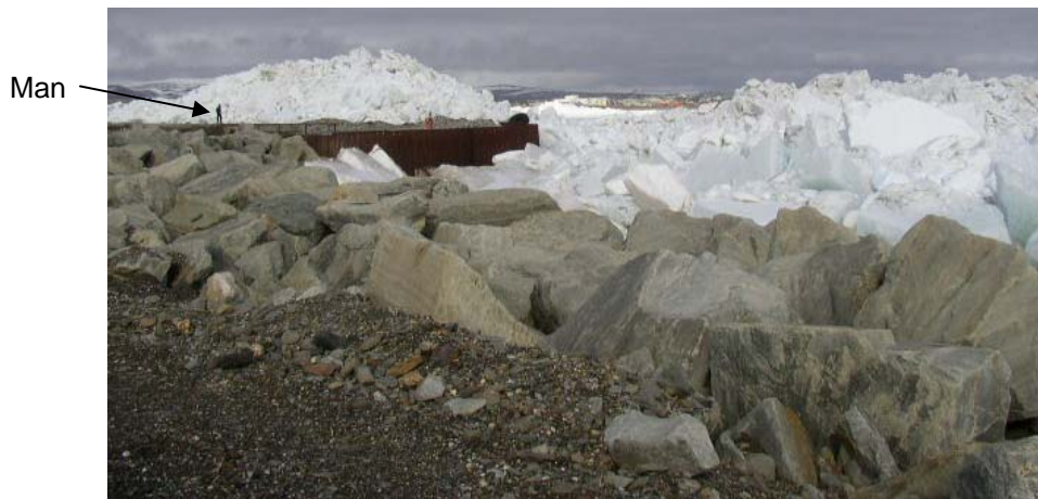
Figure 11. Man Standing on Open Cell Dock Overtopped with Wind-Driven Sea Ice, Nome, Alaska
