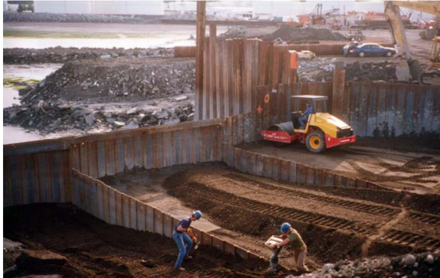
Figure 9. Open Cell Being Backfilled
